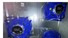
New energy efficient EC plug fans
