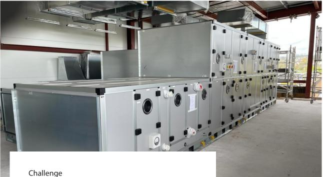
The project timeline required the AHUs to be built and positioned in place prior to the roof and walls being completed at the new hospital building, so VES were required to closely liaise with Totus on timing the deliveries in line with the crane lift.
