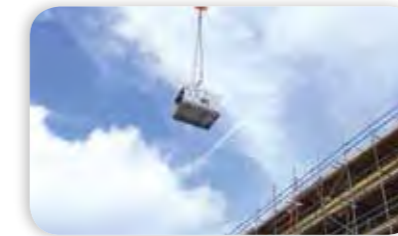
Offloading and Site Positioning
