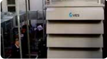
Installation of the large AHU
