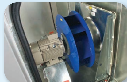
New energy efficient plug fans
