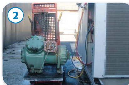
2 Compressor removed from unit
