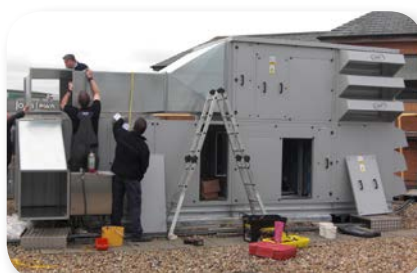
Sectional installation of VES AHU
