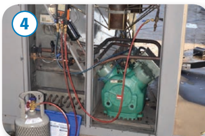
4 Unit charging and testing
