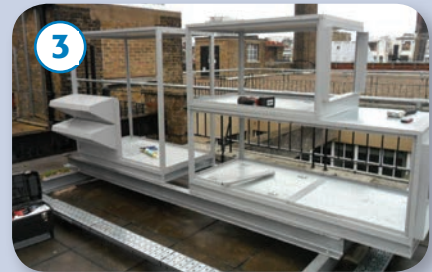
Casework being assembled
