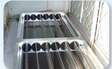
Replacement dampers installed
