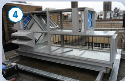
Unit components being installed
