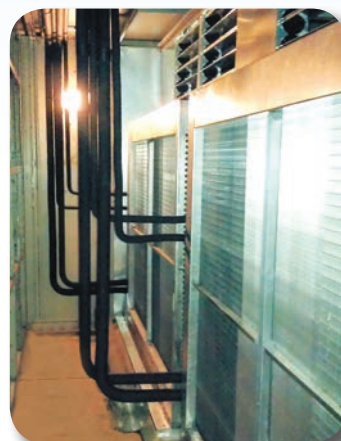
New coils installed
