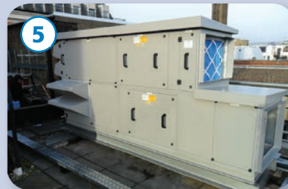
Unit fully installed
