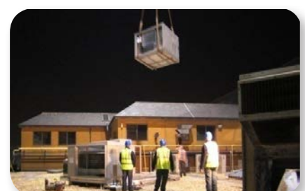
VES AHU craned into position
