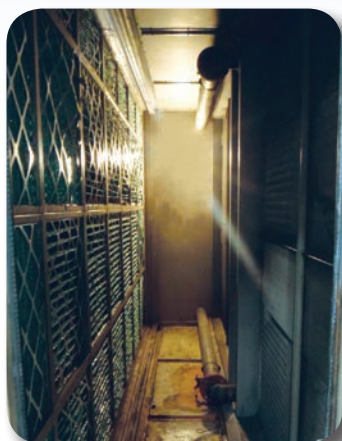
Unit before with old coils in situ
