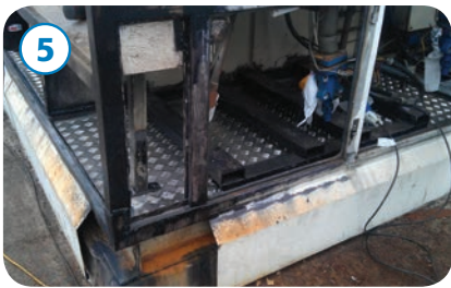
Treating corrosion and chequer plating of floor
