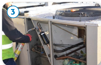
3 Brazing new filter dryer
