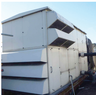
Unit condition before
