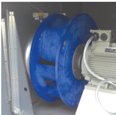
After - new energy efficient plug fan
